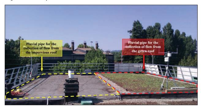
Fig. 2. Representation of the green roof and the impervious roof with the bituminous membrane
